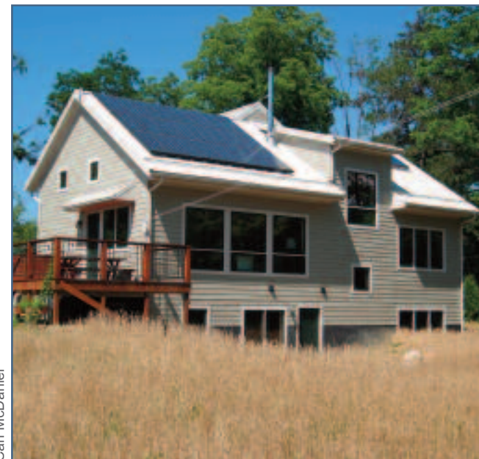
Above: South and western façades show most windows on south façade. PV panels are on west side of south roof and evacuated-tubes of hot-water system are on east side. Deck faces west and in foreground, out of sight, is the below-grade, south-facing sun patio.
